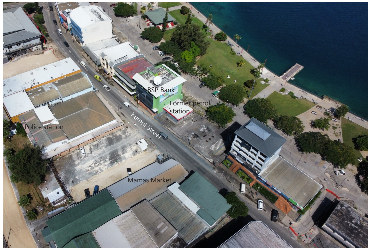
Existing view of the Town Square site
