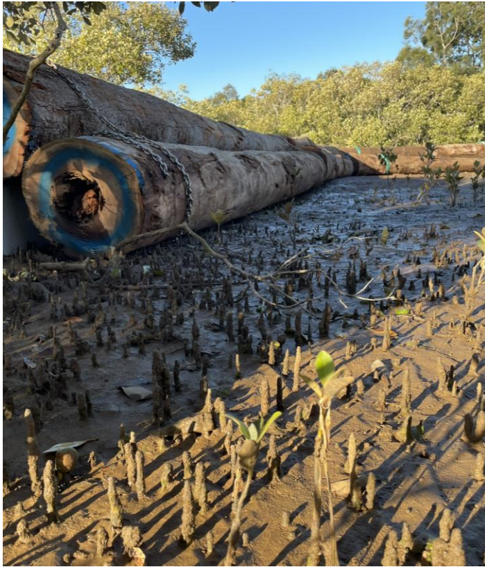
Figure 13: Log fillet offering toe support and mangrove recolonisation, Moreton Bay, Aus.(Daniel Rodger 2025)
