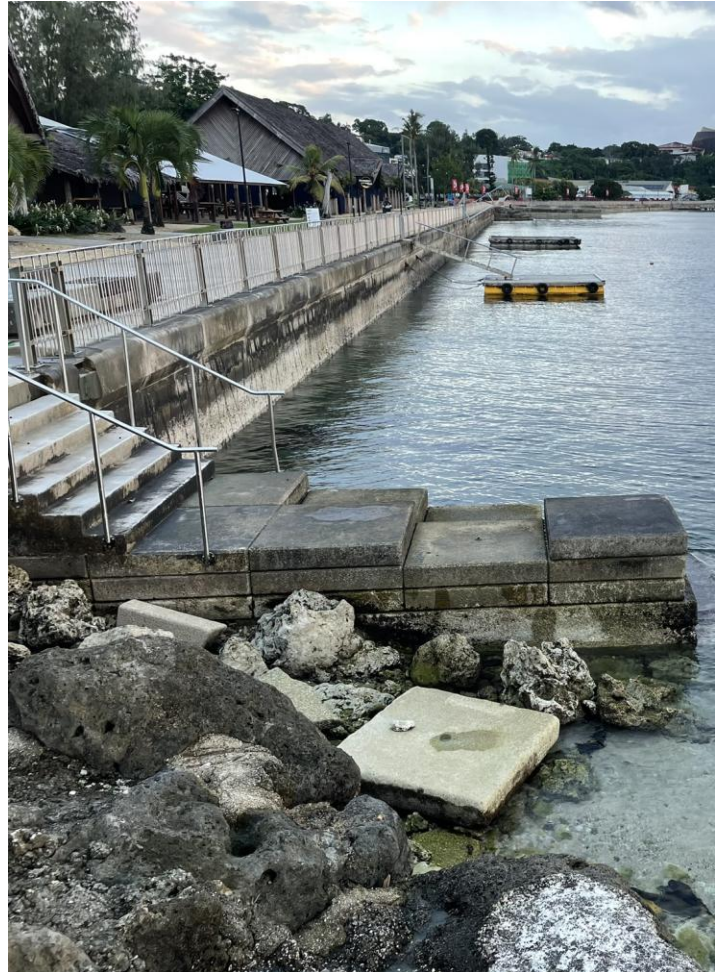
Figure 5: Port Vila seawall
