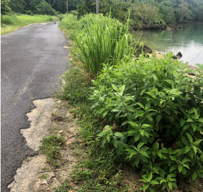
Figure 7: Lack of kerb and guttering or stormwater controls along roads adjacent to Fatumaru Bay.
