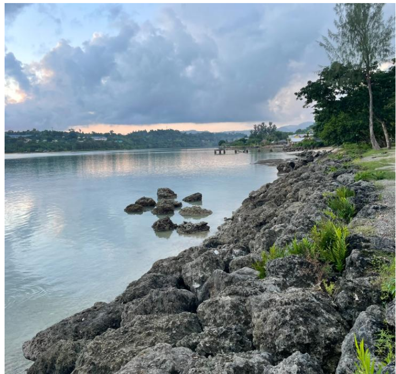
Figure 14: Port Vila northern rock revetment
