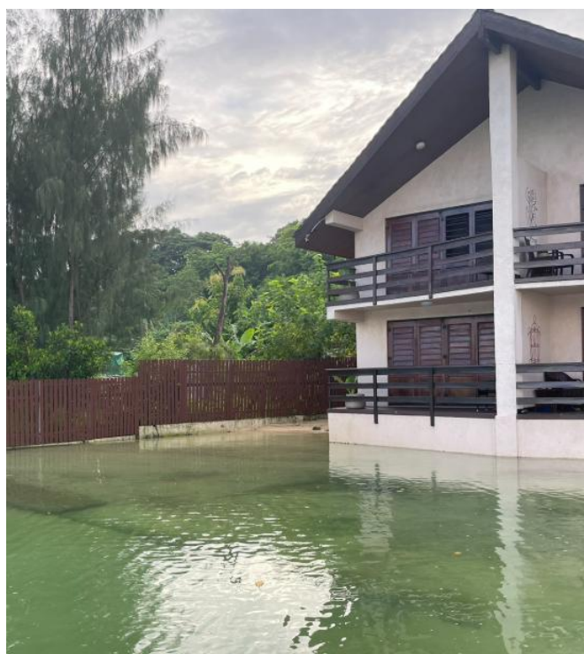
Figure 19: Fatumaru Lodge during a high tide
