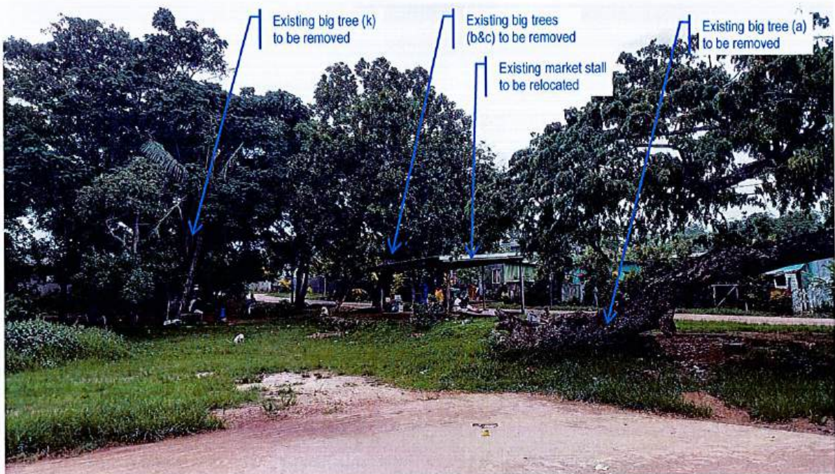
Plate 7: Existing trees within the construction area to be removed.
