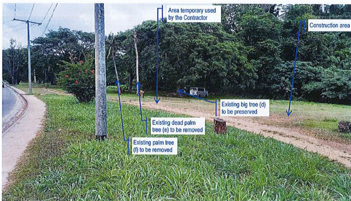
Plate 19: Existing trees outside the construction area to be kept.
