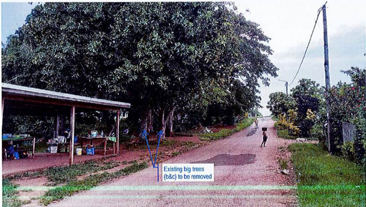
Plate 8: Existing trees within the construction area to be removed.
