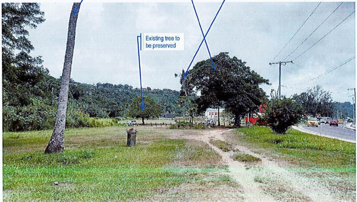
Plate 18: Existing big tree in front of the construction area to be removed (opposite view)
